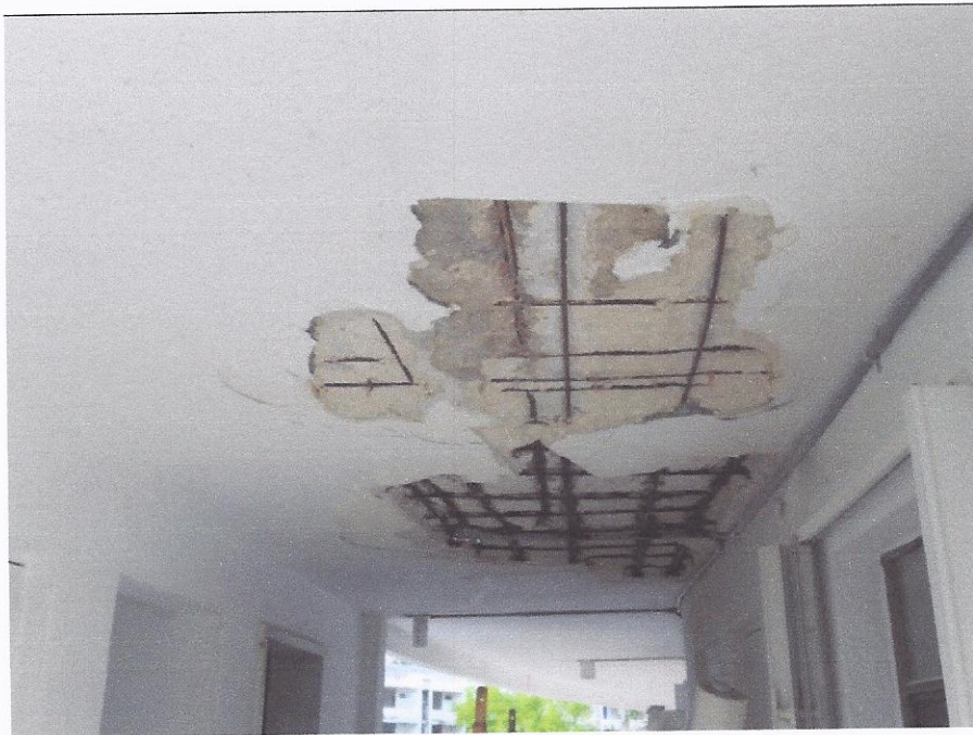
Repairs underway on 2 nd level walkways-west end near elevator-November 2012
