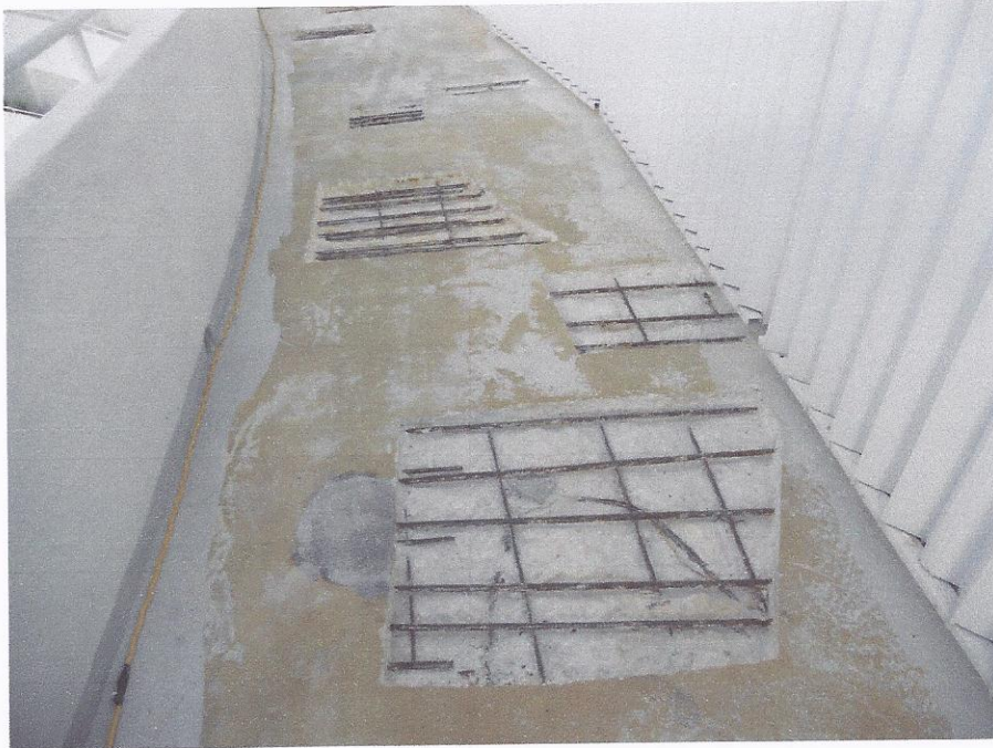
Repairs underway on unit 81 November 2012-typical of expectations
