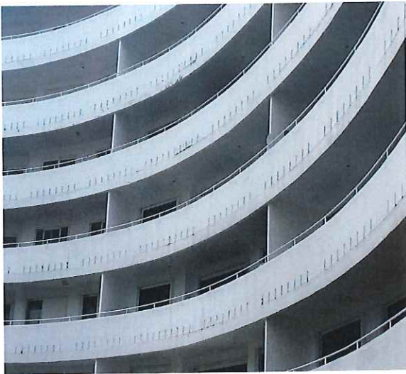
Photo#15 illustrating severe concrete crack defects at the southern CMU balcony rails.
